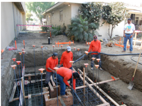
Pouring the concrete while Deputy Inspector Jose Sigala observes the pouring.
